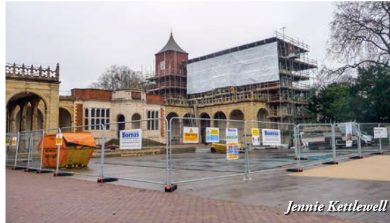
Holland House under repair
