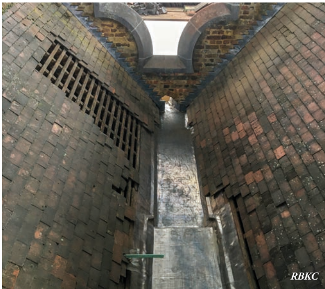
New lead gutter lining on the east wing roof
